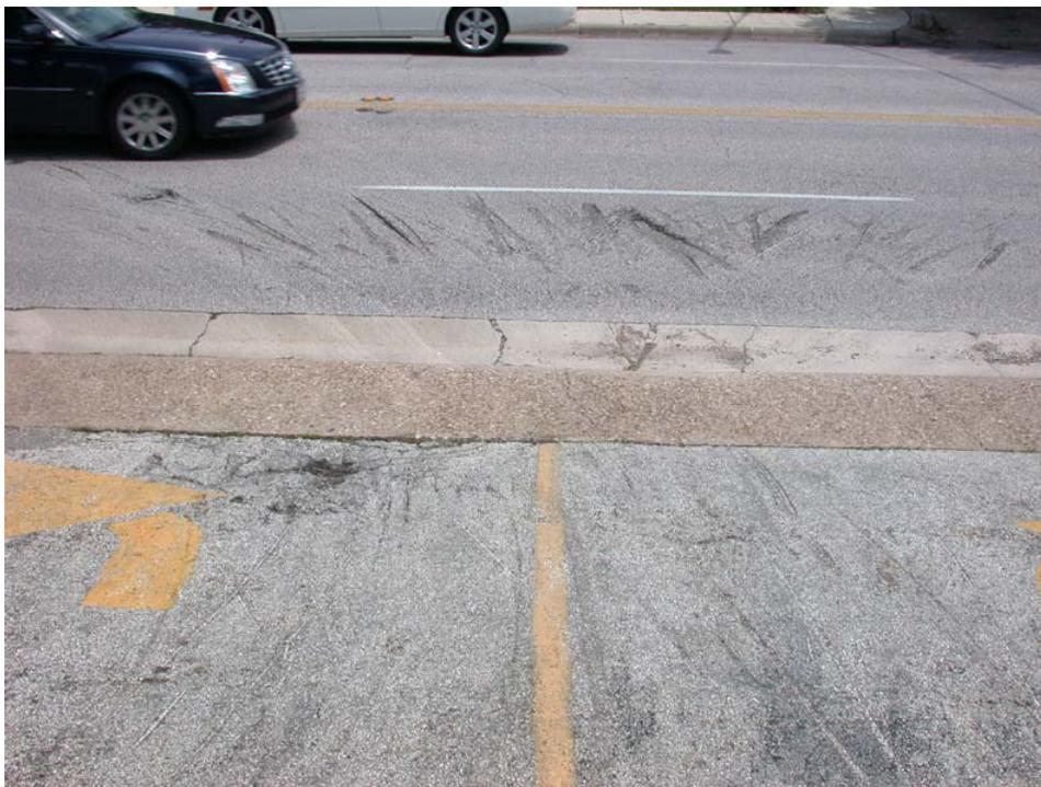
EXHIBIT 10 Example of a Driveway with Visible Vehicle Underside Scrape Marks
