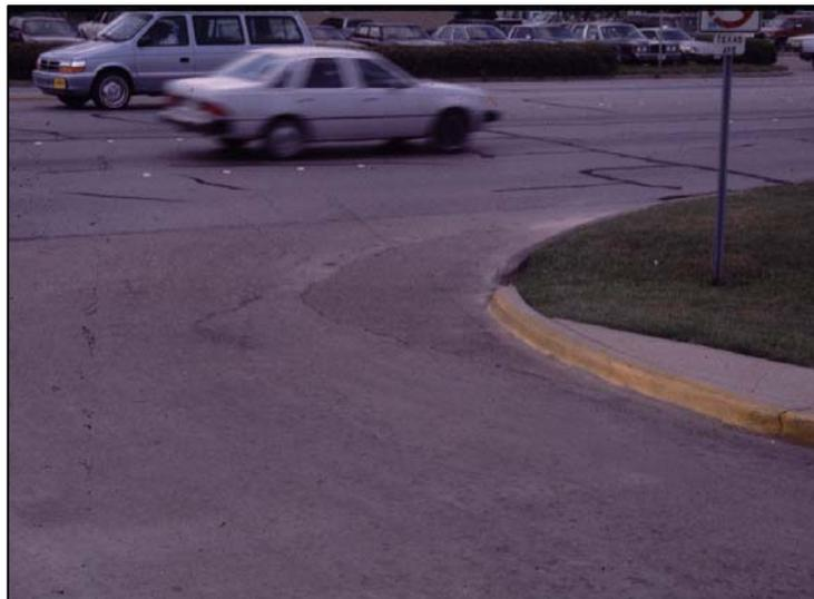
**Exhibit 6: Access Connection Was Reconstructed to Accommodate the Physical Characteristics of a Right-Turning Passenger Car**
