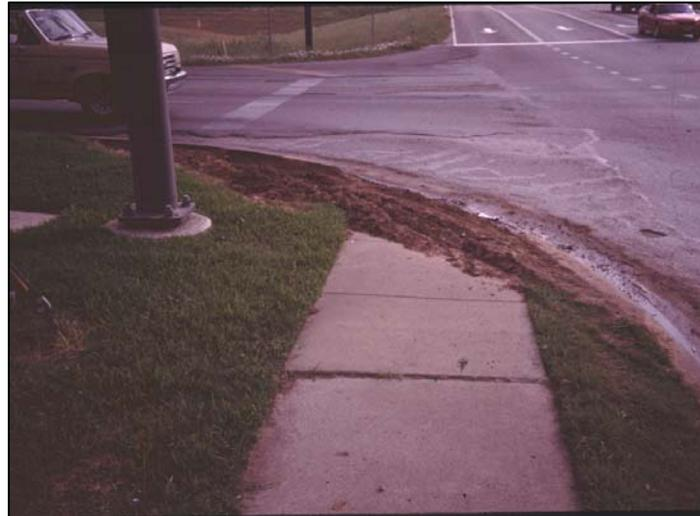
**Exhibit 5: Inadequate Radius Results in Damage to Curb Return and Sidewalk**
