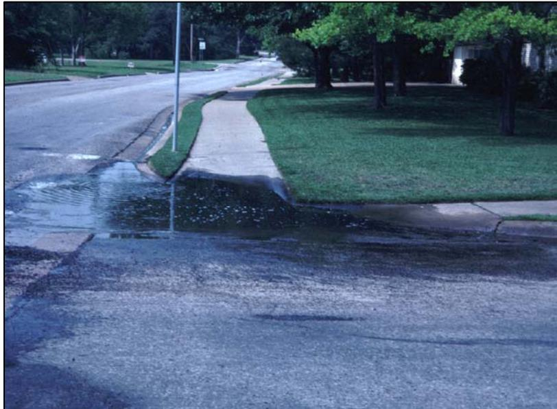
**Exhibit 8: Poor Intersection Design Resulted in a Drainage Problem**
