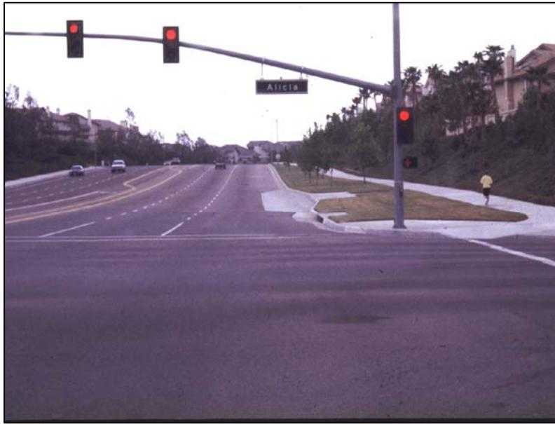
**Exhibit 18: Example of Mast Arm Mounted Sign to Aid in Intersection Visibility/Identification**
